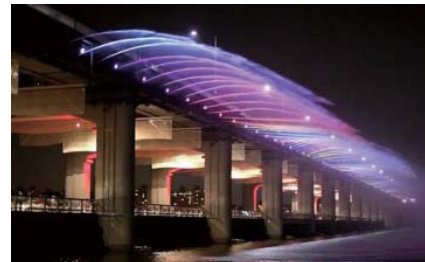
Banpo Bridge Analysis (Daewoo Engineering) Final Design(Considering the additional load of the fountain facility)
