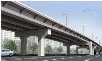
Main Line Overpass Juam Bridge
