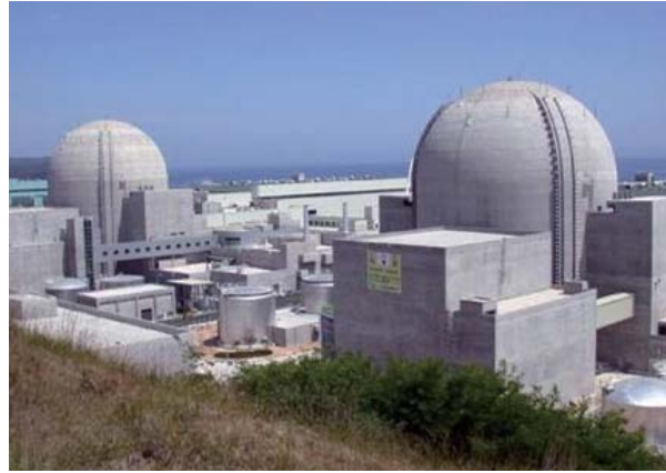
Uljin #3, 4 Nuclear Power Plant (Korea)
