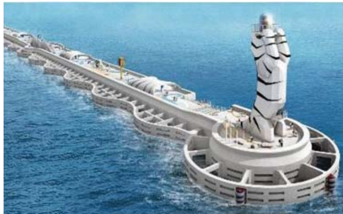
Yeongil new port breakwater project (Korea) - Length : 800m
