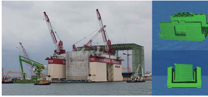
TUAS TERMINAL PHASE 1 Project (Singapore) - Caisson Self-Float, Transportation, Float-off, Towing
