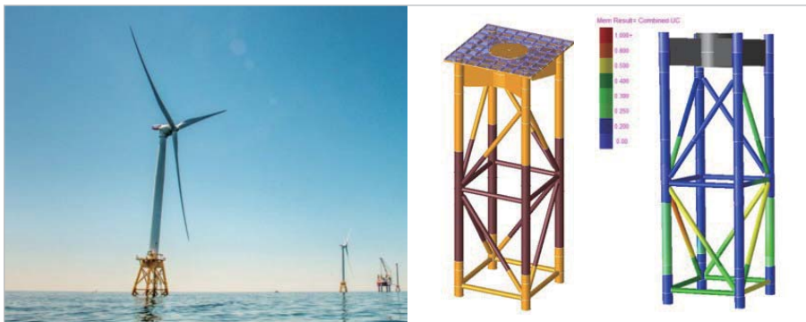
Development on integration design and construction method of the jacket structure of offshore wind turbine for cost savings of marine construction, Korea Institute of Energy Technology Evaluation and Planning (KETEP) - Integration design and construction method of the jacket substructure for offshore wind turbine to save installation cost
