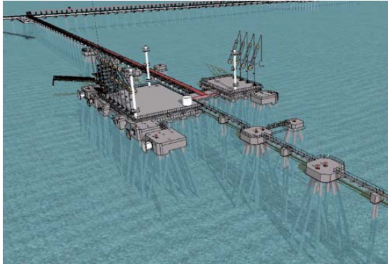
BM Energy LPG jetty project (Bangladesh) - Jetty : 1set, CBM : 4 Buoys, PLEM : 1set
