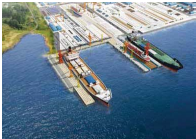
MMHE west finger pier Basic & Detail Design (Malaysia) - Quay wall : 665m, Seawall : 210m
