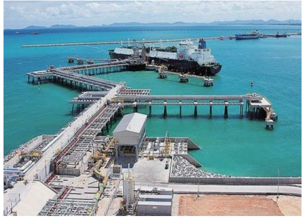
PTT LNG receiving terminal project (Thailand) - W/ P : 1set, BD: 3set, MD : 6set, Trestle : 250m - Design Vessel : 266,000m 2 Carrier
