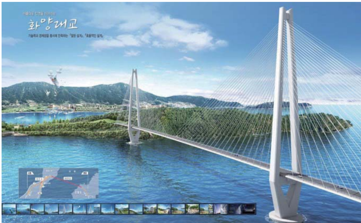
Hwayang~Jeokgeum 2 Zone (Iksan Regional Construction and Management Administration) Scope : Length = 854.0m , Main Tower Height= 170.7m , Interval = 500.0m
