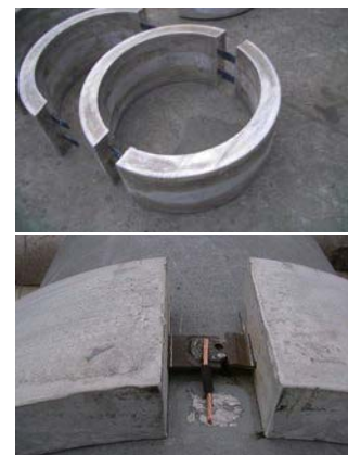
Cathodic Protection (Anode)
