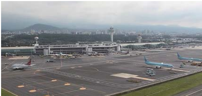
Jeju International Airport (Daewoo Engineering) Culvert, Paving, Retaining wall etc. Detail Design for Railway
