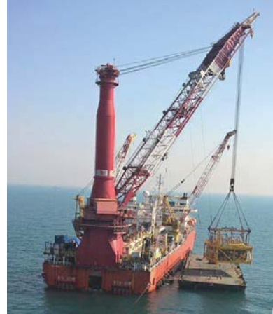
VASAI East Development (India) - Topside Installation
