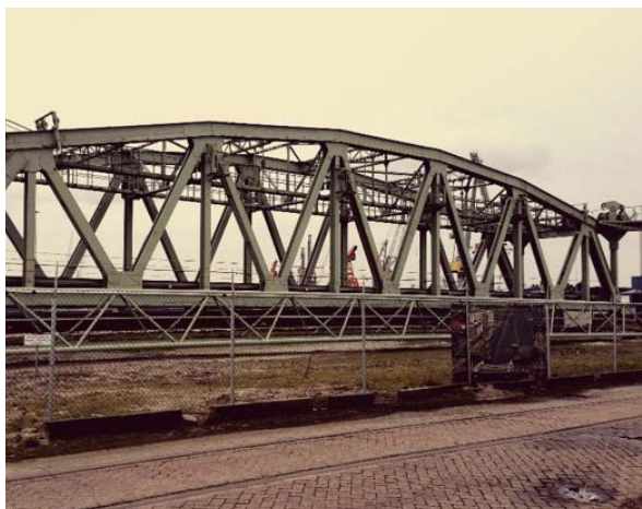
Railway Bridge and Box for Western Line (Korea) - Bridge and Tunnel Box Detail Design for Western Railway
