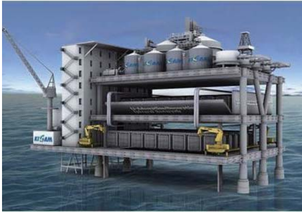
Seawater dissolved Lithium Deportation Plant
