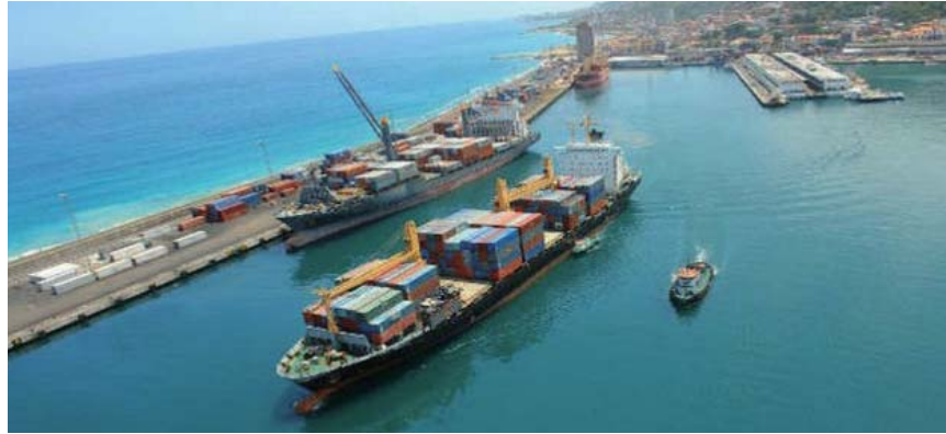
Feasibility study for multi-purpose port development project near Chittagong (Bangladesh) - Dolphin : 3 Berths, Trestle : 1,000m, Embank : 500m
